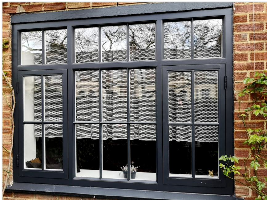
Exterior – restored multi-pane timber window finished in period colours
